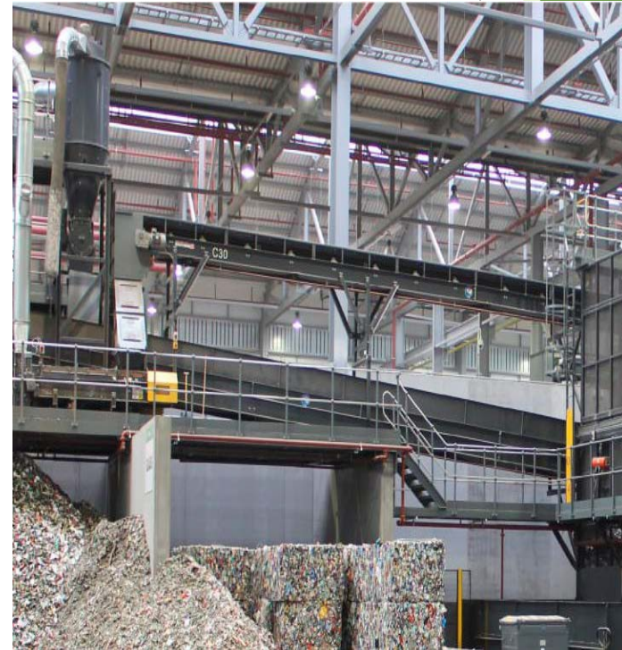
CP Glass Cleaning System
