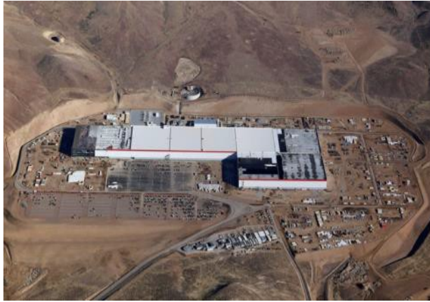
Tesla® Gigafactory One, Sparks NV
